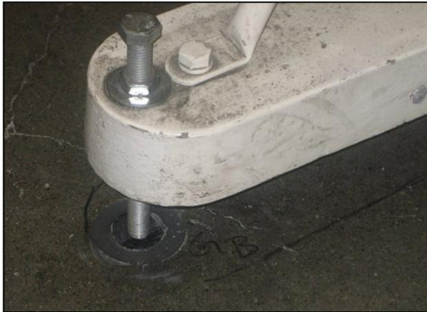
Figure 9. V-block Mounting Point (installed)
