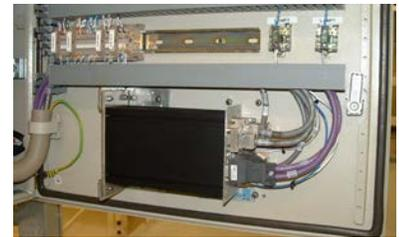
radiomatic wireless pendant and hydraulic pump as it removed the requirement of passing information between separate controllers. The controller is a Siemens CPU315-2DP with integrated Profibus. The HNC's and any other I/O connect to the PLC via this single Profibus. The total length of the Profibus network is 400M and it runs at 500kHz.
