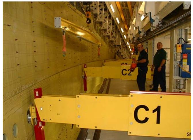
Figure 8, Panel shown during removal process. Panel is completely supported by panel loader arms and then drawn away from sub structure.
