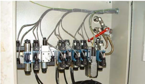
Figure 6, Hydraulic manifold typical each arm.
