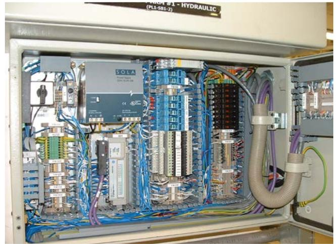
Figure 7, Electrical controls typical each arm.
